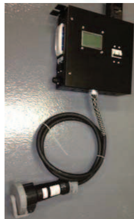
Figure 11: Busway Application for dc Distribution (Source Universal Electric)
