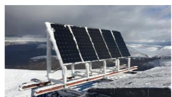
One would think that the Arctic would not be the most economic place to install a solar hybrid system. However, considering the difficult access for diesel refill, which is by helicopter only, and the long hours of sun in the summer, Eltek has made it pay off.
