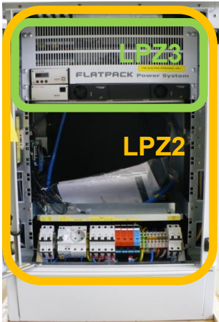
Figure 2-2 Lightning protection zones example in an Eltek outdoor cabinet solution
